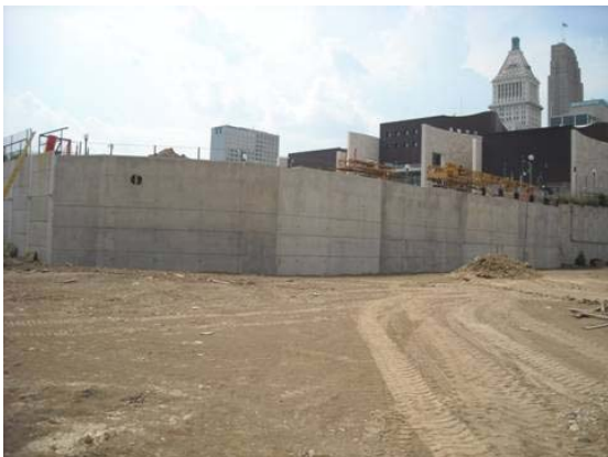
Walnut St. retention wall complete with concrete facing. Shear wall construction.
